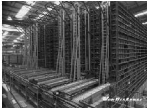
Figure n°1.9: Mini-load system (courtesy of Vanderlande)
