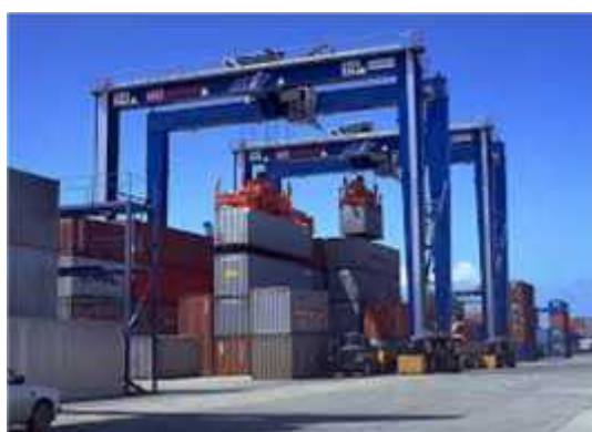
Rubber-tyred Gantry Cranes (RTGCs).
